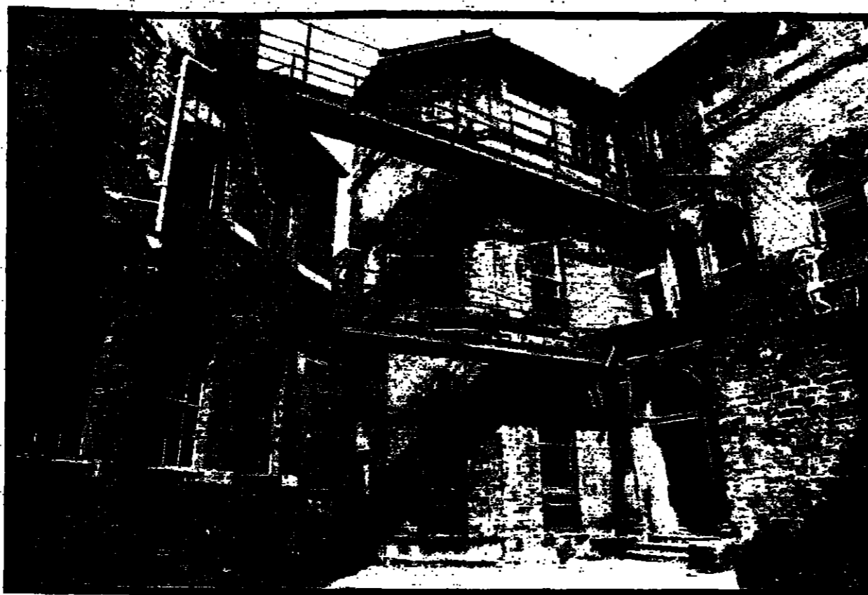
Cornish Place, Sheffield: once a cutlery factory, the Grade II building will be transformed into homes and work units
